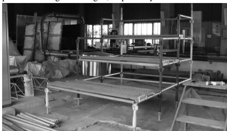
Fig. 2. Front view of temporary steel grandstand considered in the study
