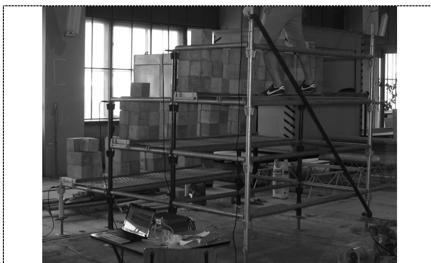
Figure 1. Steel temporary grandstand with typical diagonal stiffener.
