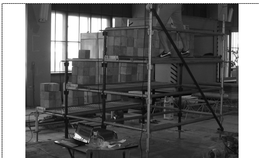
Figure 1. Steel temporary grandstand with typical diagonal stiffener.
