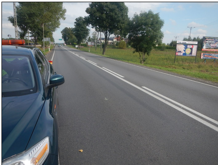
Figure 5. Test section SMA 11-R as seen west direction
