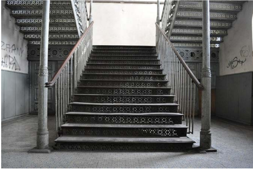
Fig. 1. Cast iron staircase: general view.
