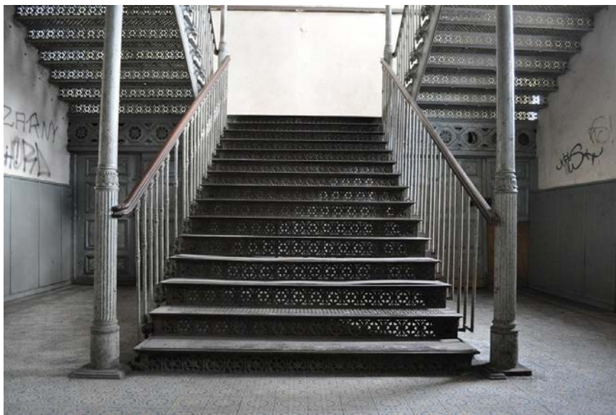
Fig. 1. Cast iron staircase: general view.
