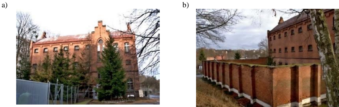
Fig. 1. Building of the garrison arrest: (a) from the south, (b) from the north with the perimeter wall encircling the prison yard.
