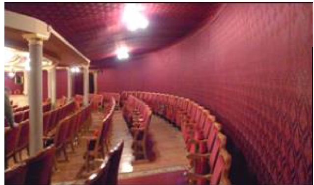
Fig. 8. The underbalcony space in the Lviv Opera House hall prior to installing the sound diffusing structures. The walls and ceiling were covered with a textile tapestry.
