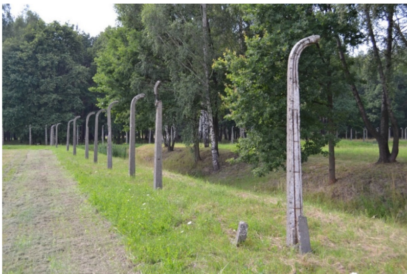
Fig. 2. Some poles need still renovation.
