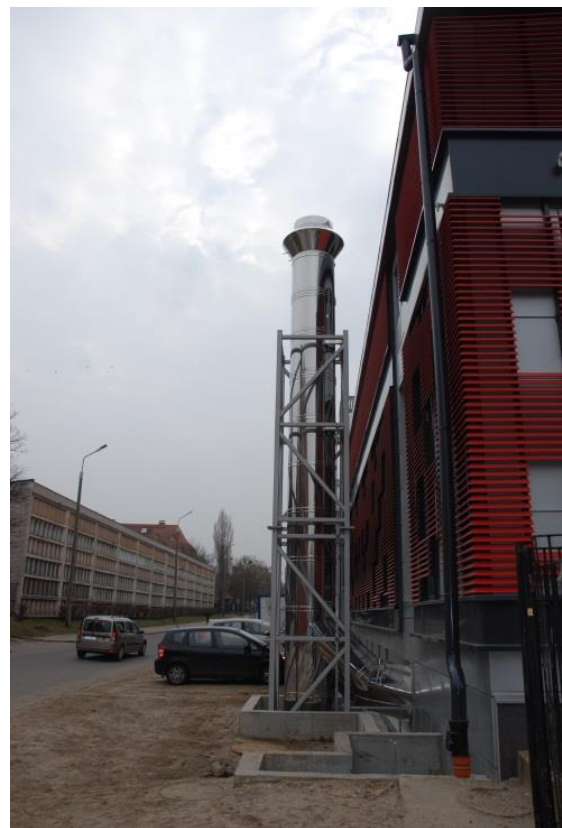
Img 2. Air inlet (a) and exhaust gas outlet (b) of the turbine engine
