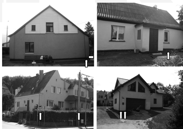
Fig. 1. Buildings tested for traffic-induced vibrations (arrows indicate the locations of vibration sensors)
