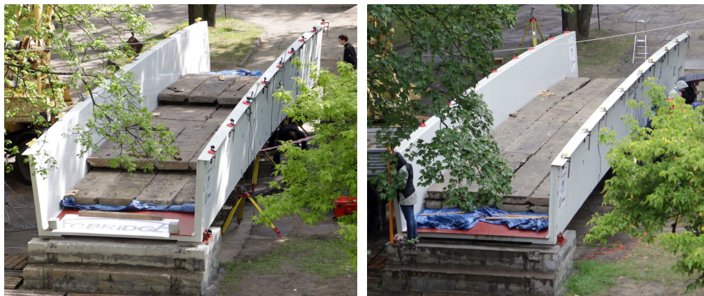
FIG. 2. Footbridge loaded during tests U1 (left side) and U3 (right side).
