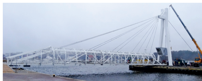
Fig. 1. Rotating footbridge for pedestrians over the Ustka port channel (configuration W1a)
