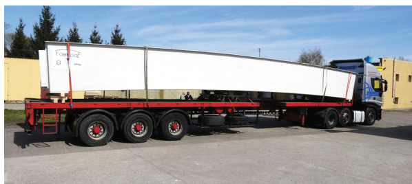
Fig. 11. Transporting the footbridge span
