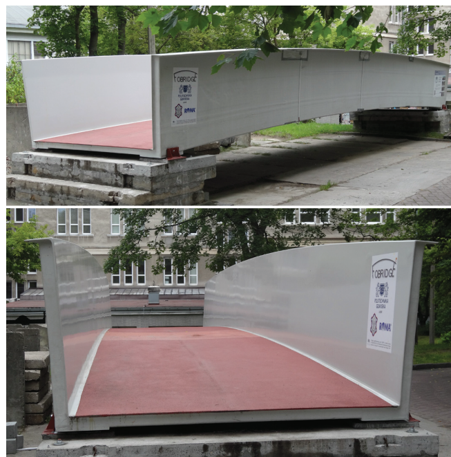
Fig. 3. Composite span of the FOBRIDGE walking and cycling bridge
