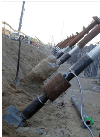
Fig. 9. Installation of the rod Z2 segment fitted with gauges
