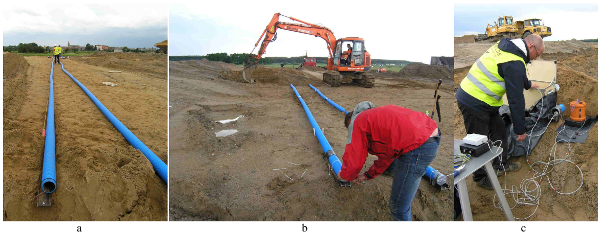
Fig. 8. a, b. Installation of tubes; c. First measurement after tubes backfilling
