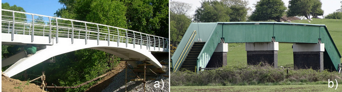
Fig. 5. a) Arch footbridge in Moscow, Russia (Source: www.apatech.ru), b) Bradkirk Bridge in Kirkham, UK (Source: own image)
