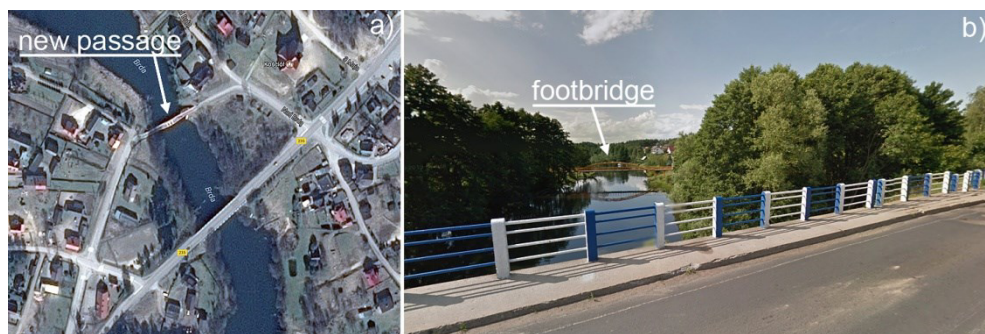
Fig. 3. Footbridge in Męcikał: a) location, b) view from the road No. 235. Source: www.google.pl/maps .
