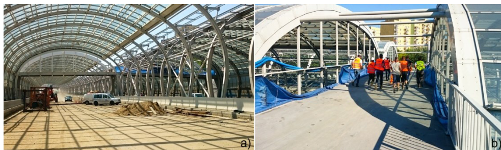
Fig. 6. Footbridge in Warsaw over S8 express road during load test.
