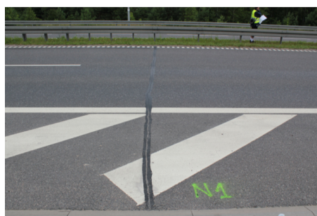
Figure 3. Repaired low-temperature crack.
