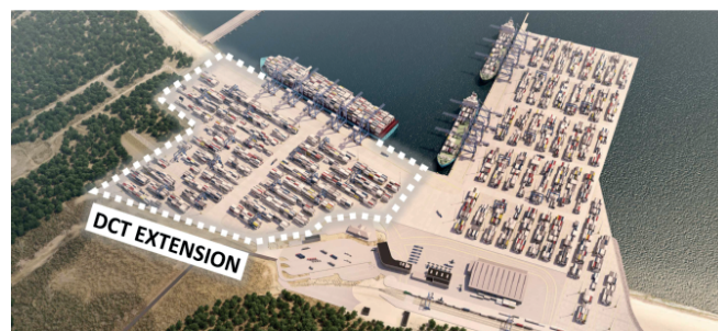
Fig. 3. Bird view of the new quay wall and container storage yards (acc. DCT Gdańsk S.A.)
