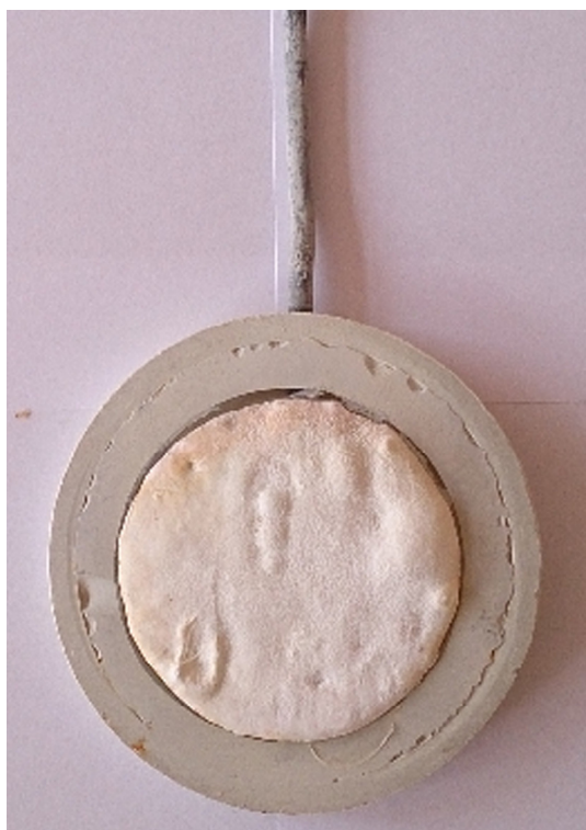
Fig. 10. Specimen covered in calcareous cathodic products after 9 months of exposure.
