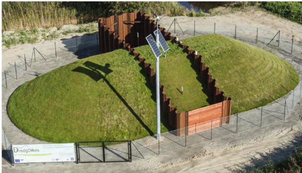
Fig. 1. Test dike in Trzcińsko - near Gdańsk [8].
