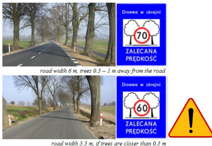
Fig. 5. Recommended speed on sections with trees close to the edge.
