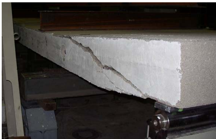
Figure 8. A typical failure mode of the wall components on the example of specimen 2.2
