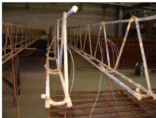
Figure 4. Steel lattice girders prepared to be built in the tested wall components of the improved structure (the second and third types). Installed strain gauges with electric wires are visible
