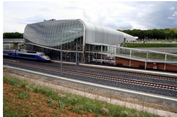
Figure 2. Belfort-Montbéliard TGV (D.Zaluski). Distinctive form of the tube made of laminated wood covered with galvanized steel helps to reduced energy consumption.
