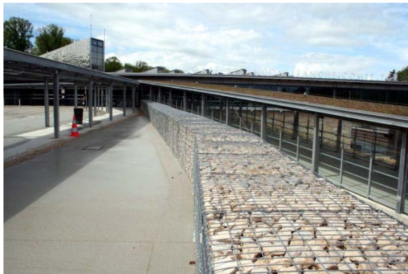
Figure 1. Besancon FC TGV (D.Zaluski). Additional thermal insulation delivered by its green roofs and the shape of the building itself.
