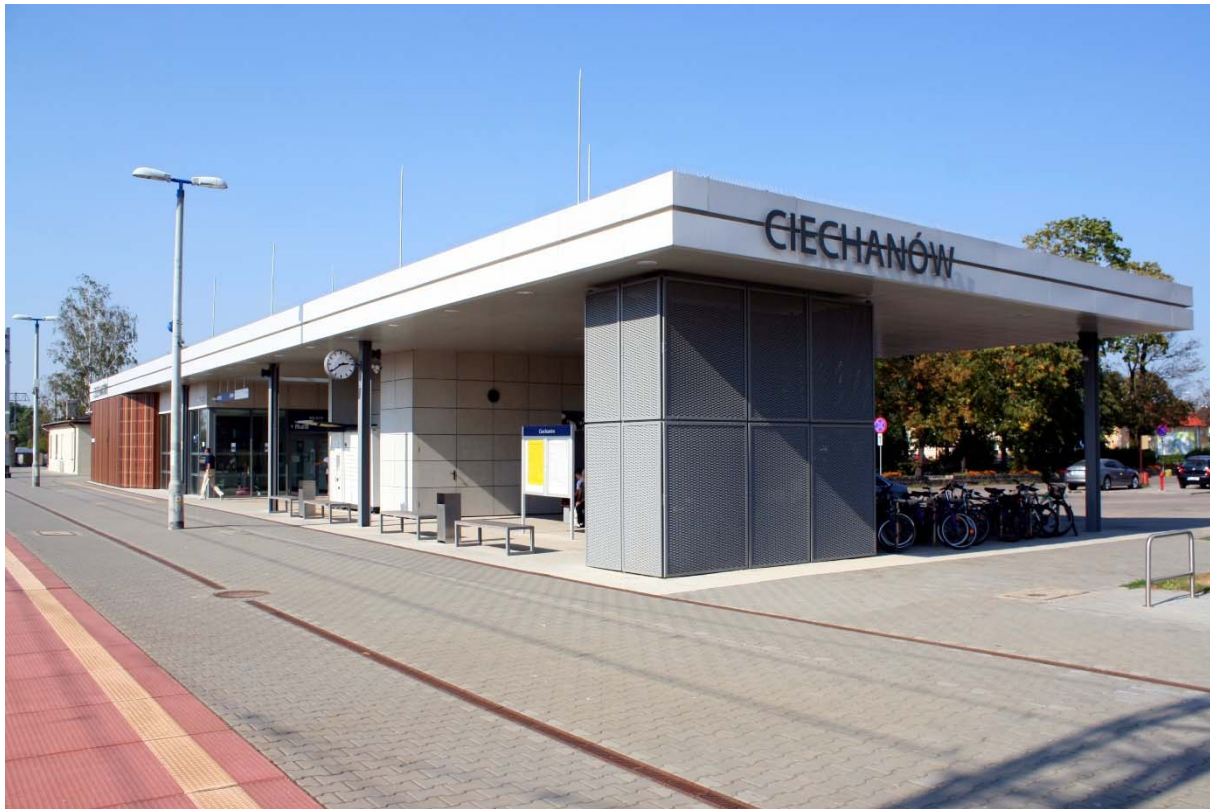
Figure 5. Innovative Railway Station in Ciechanów (D.Zański). A seasonal waiting room shaded and well protected from the rain by a large field of the extended roof. Also a place for bicycle racks, vending machines, storage lockers and ATMs
