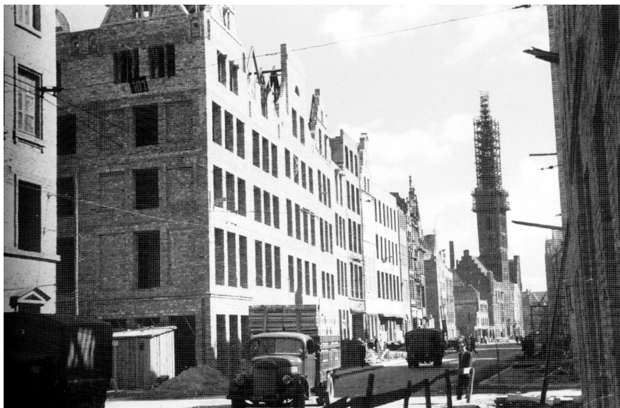
Figure 1. Ulica Długa ( Langgasse ) during rebuilding (Collection of the Faculty of Architecture, Gdansk University of Technology, ca. 1950).
