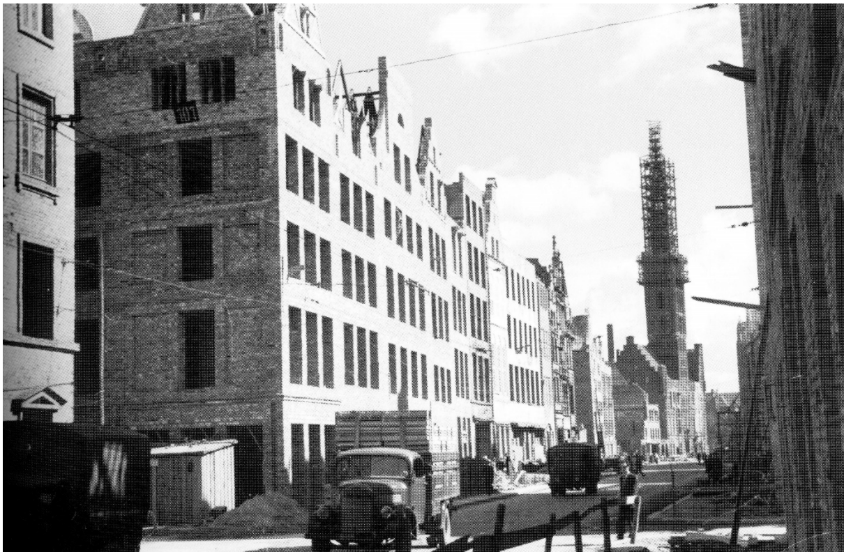
Figure 1. Ulica Długa ( Langgasse ) during rebuilding (Collection of the Faculty of Architecture, Gdansk University of Technology, ca. 1950).
