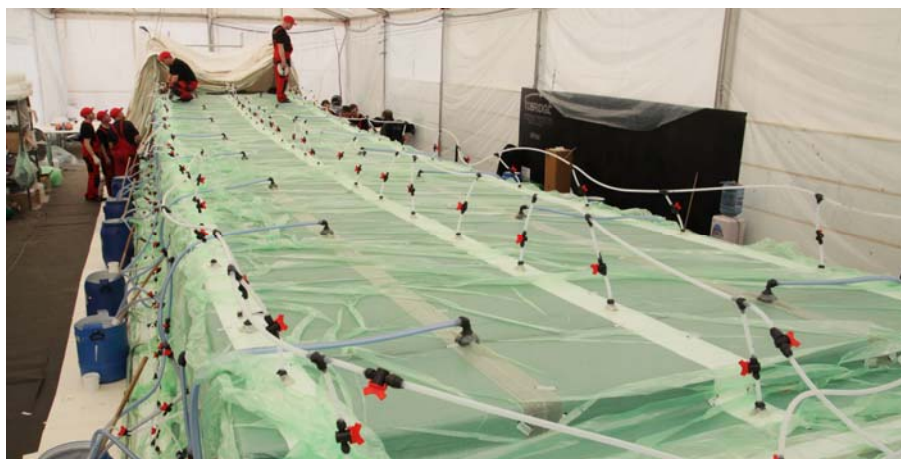
Figure 3. U-bridge footbridge production process
