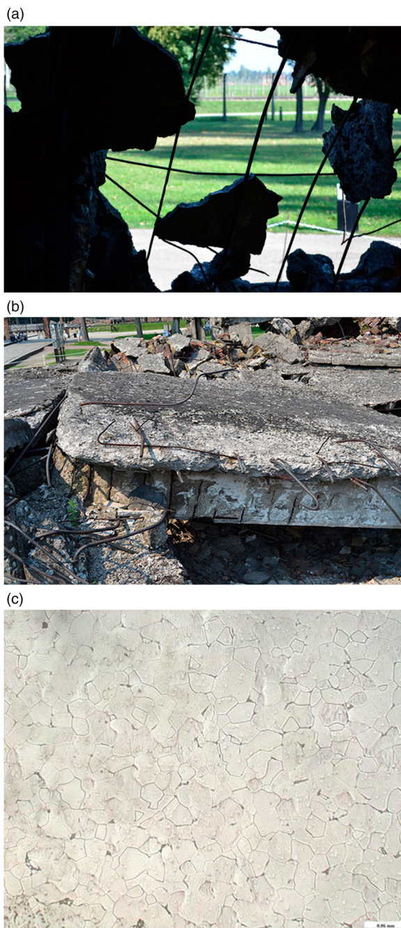
Figure 5 Uncovered reinforcing steel bars of the ruins of the crematorium II in Auschwitz II-Birkenau (A), a ceiling of the gas chamber of this crematorium (B), and the metallographic structure (grainy ferrite and very small amounts of perlite, several non-metallic inclusions, magnification 200 \times ) of the reinforcing bar adopted from Gotkowski & Jachym, 2014 (C).
