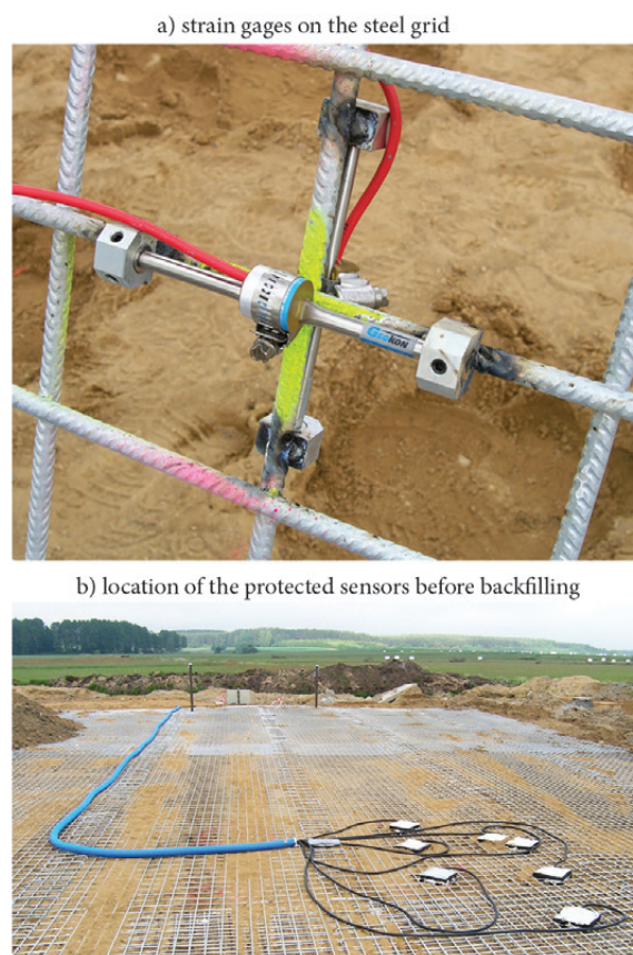
Fig. 6. Measured points on steel grid
