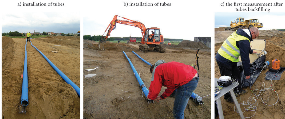
Fig. 8. Embankment settlement measurement by hydrostatic levelling
