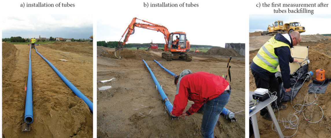
Fig. 8. Embankment settlement measurement by hydrostatic levelling
