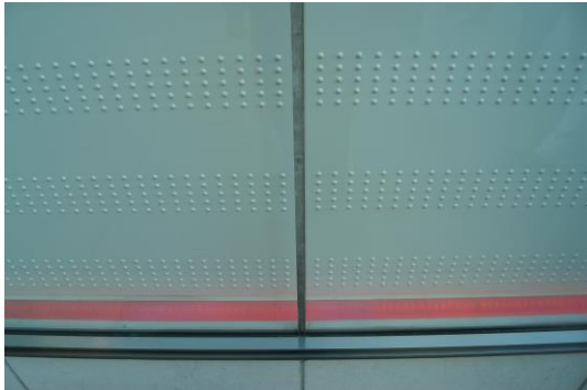
Fig. 15 Matsuya Ginza – detail of the curtain wall
