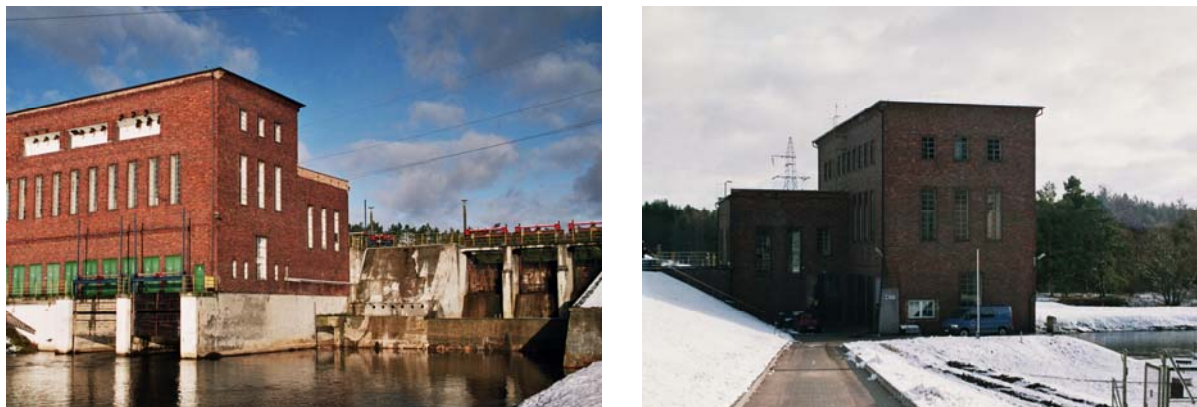
Figure 6. Jastrowie power plant. On the left: tailwater view; on the right: headwater view
