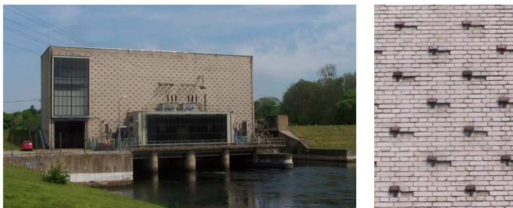
Figure 8. Tryszczyn power plant (1956-62), river Brda. On the left: tailwater view; on the right: brickwork detail
