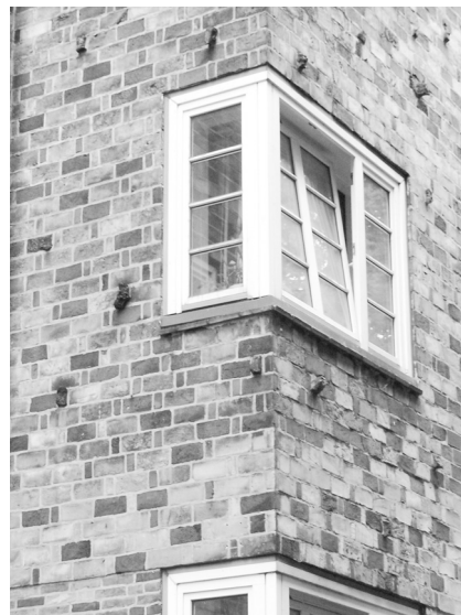
Photo 2. Detail of the clinker façade – Helmoltzstrasse multifamily house
