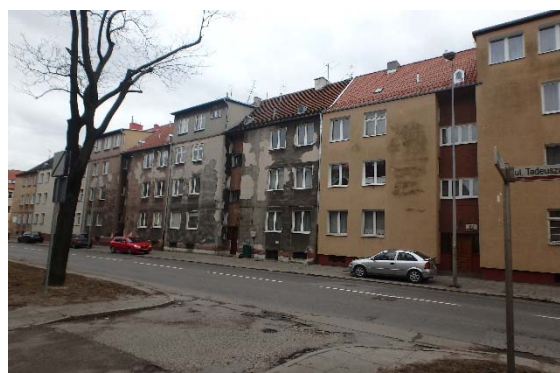
Figure 5. Back in the middle portion of the building [10]
