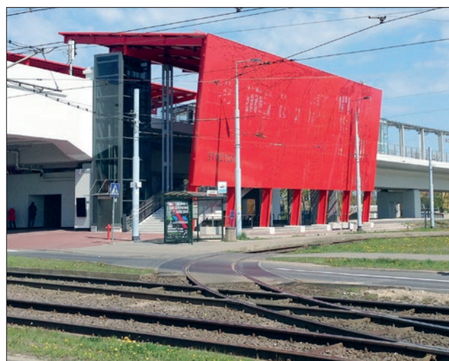
Figure 6 Metropolitan Railway Station – innercity intermodal junction
