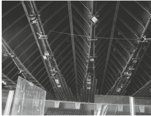
Fig. 10 Structure of the roof of “Olivia” Sports Arena in Gdansk, Poland
