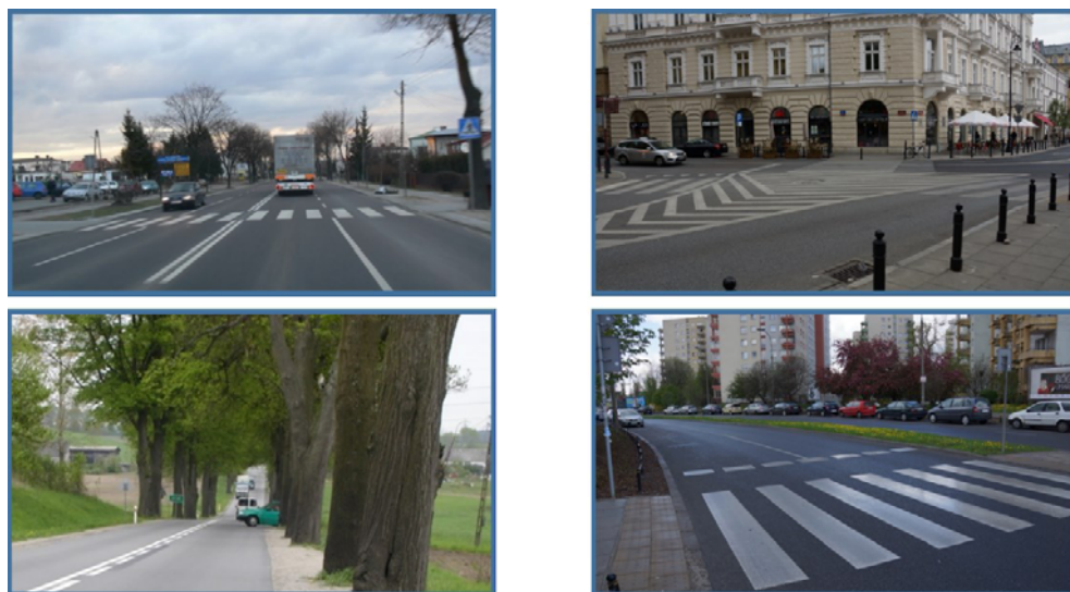
Fig. 3 Examples of road defects.
