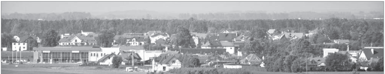
Figure 4: Residential fabric in Chwaszczyno with service buildings (photo: Grzegorz Peczek)
