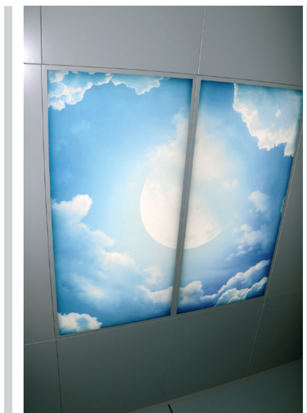
Figure 7. The LED Skylight as innovative ceiling finishing in treatment rooms in hospital, 2016, Photography: A. Gębczyńska-Janowicz
