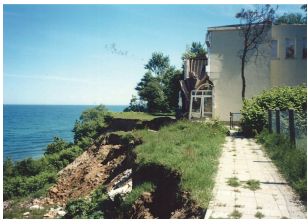
Fig. 2. The leisure centre "Horyzont" situated on the edge of an active cliff and damaged in 2002. (photo courtesy of W. Subotowicz)
