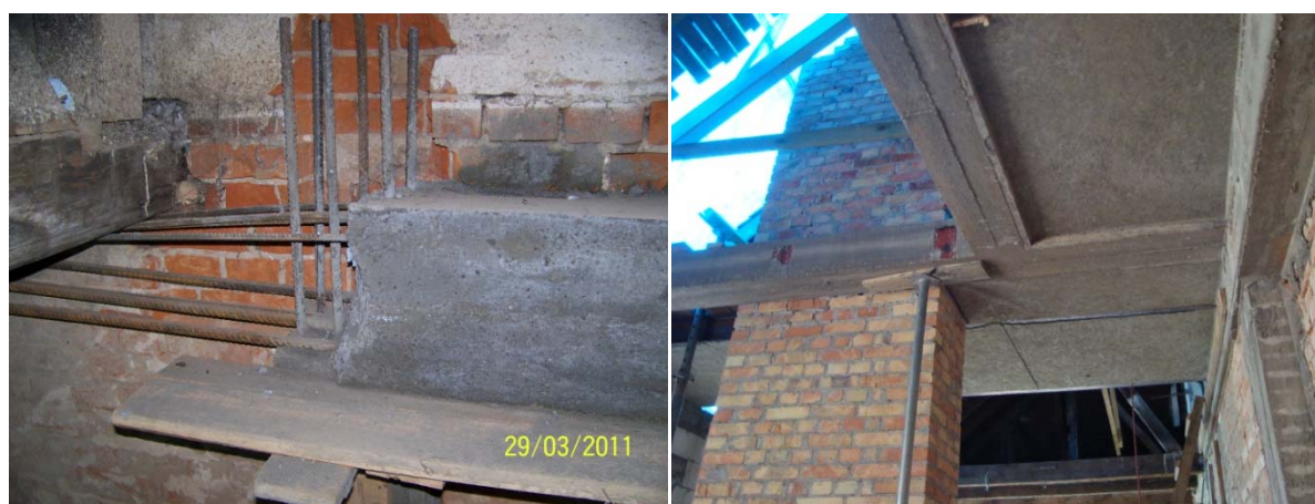
Figure 2. Example of reinforced concrete construction
