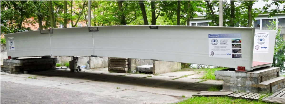
Fig. 1.3 Full scale research object of pedestrian bridge, developed, under FOBRIDGE project at Gdańsk University of Technology, Gdańsk, Poland.
