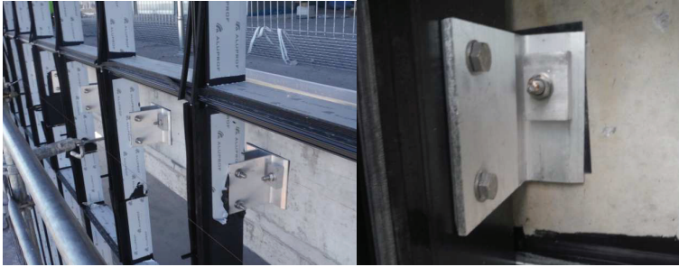
Fig. 1. Mullion-transom wall system – aluminium profiles and brackets
