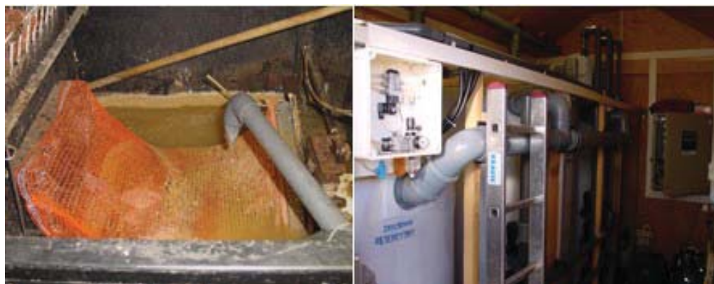
Fig. 2. Biovac® wastewater treatment plant at West Spitsbergen a) bag screen , b) retention tank [10]
