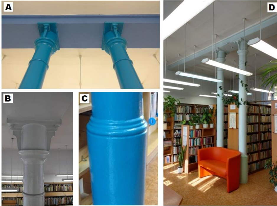
Fig. 3. Cast iron columns in the building of the former financial office in Kwidzyn: A - view of the beam's double support, B – detail of the column capital, C - base detail, D - general view.
