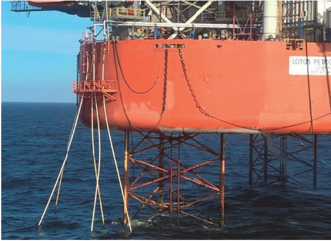
Fig. 14. CT 4" pipes operating in the water injection system on the LOTOS Petrobaltic platform
