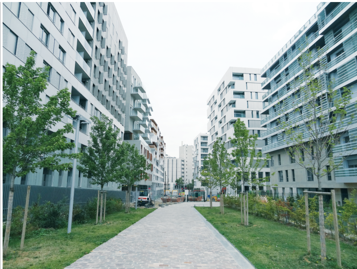
Figure 4. ÉcoQuartier Clichy-Batignolles, Paris, Parc Martin Luther King: architectural variety, Photo: M. Trojanowska
