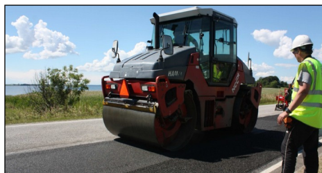
Figure 8: Construction of the first Danish full scale test track in Kalvehave (Kalvehave I): the fresh PERS mix in front of the gussasphalt paver was first spread manually (left hand side) and then compacted (right hand side)
