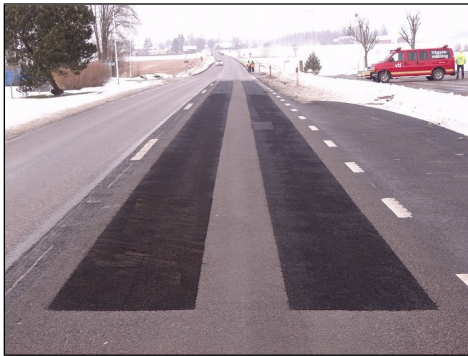
Figure 13: Swedish full scale test tracks in Sjögestad in February 2016, i.e. 1,5 years and two winters after construction. The Sjögestad II surface with the PERS prefab panels (applied only in both wheel tracks) can be seen on the foreground. Note some scars by the snowplough and some raveling. The slightly lighter coloured PERS surface in the background the original in situ constructed PERS test track (Sjögestad I)
