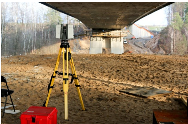
Fig. 10. Laser scanner Leica P30 station.
