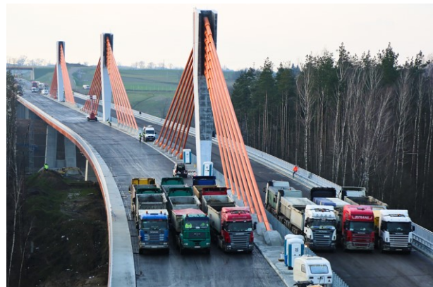
Fig. 5. Full ballast loading during U45 setting.
