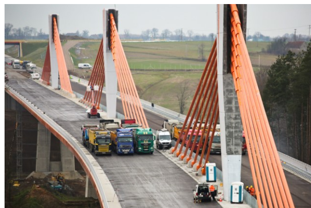
Fig. 4. Full ballast loading during U34 setting.
