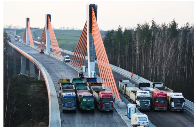
Fig. 5. Full ballast loading during U45 setting.
