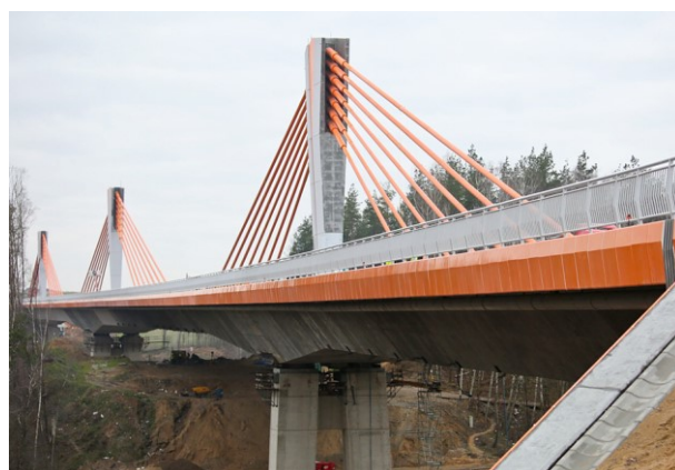
Fig. 1. Side view of MS-3/DK-16 bridge.
