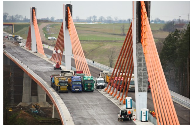
Fig. 4. Full ballast loading during U34 setting.
