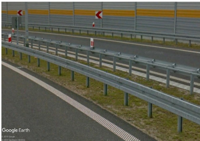
Fig. 1 N2/W4/A steel road safety barrier on A1 highway in Poland, credits: Google Earth.
