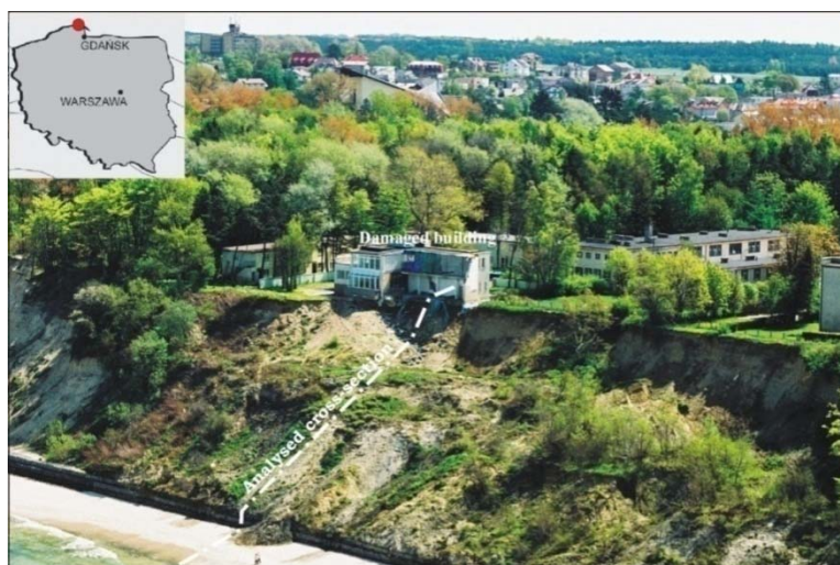
Figure 1. General view of the landslide on the cliff
