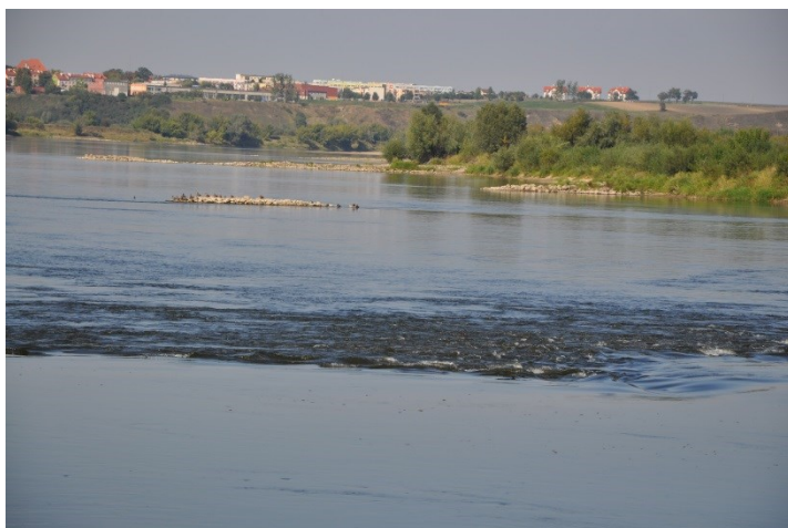
Fig. 3 Regulatory buildings in the Vistula delta [fot. P. Jerzyło]
