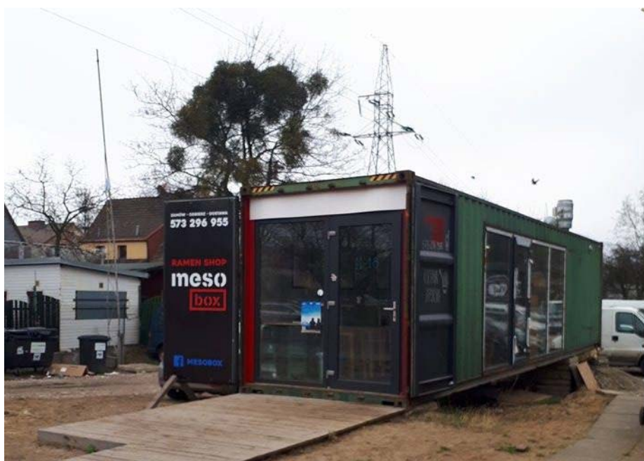
Figure 1. Small restaurant made out of 40' HC shipping container
